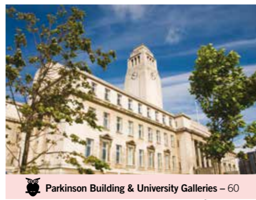
Parkinson Building & University Galleries - 60
