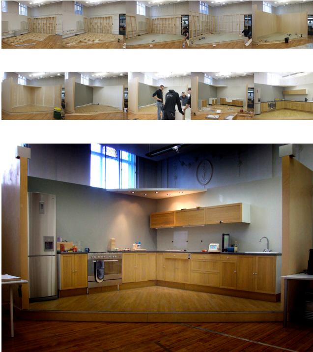
Figure 1. The Ambient Kitchen is a lab-based high fidelity pervasive computing prototyping environment. The kitchen is situated in the main research space in Culture Lab, Newcastle University and uses modified IKEA units and standard laminate flooring installed within a wooden structure (see top figures). Significant care was taken that the underlying technology is not apparent to the people using the kitchen – even the wall projection is achieved using “up-lighter” style projection onto mirrors below the overhead cabinets.
