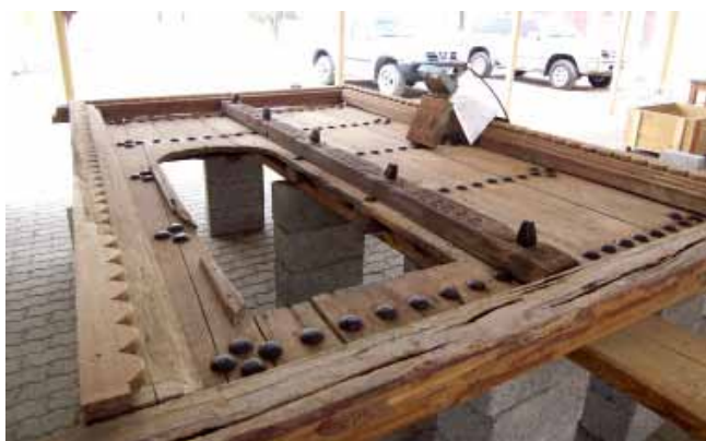
Figure 29 - Treating a historic door against termite infestation. The beautiful door comes from the house of the late Sheikh Mohammed Bin Khalifa al Nahyan in Al Ain (Photograph: Ege Yildirim).
