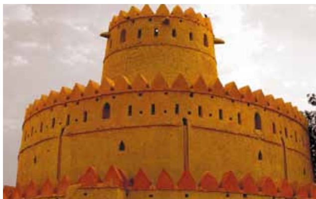
Figure 23 - View of Jahili Fort in Al Ain (Photograph: ADACH).
